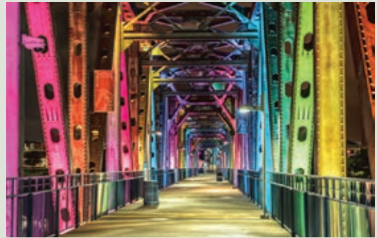
Junction Bridge Pedestrian Walkway
