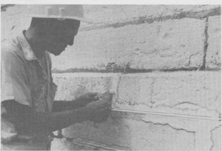
Fig. 8. The mason has tooled the joint with his pointing trowel and is now removing excess mortar from the face of the stone.
