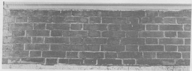
Fig. 5. A good example of proper spot repointing of brickwork, where the mason has paid due attention to the color and texture of the original pointing material. Excess mortar from each replaced joint has been carefully removed from the corners of the brick with a knife blade to closely approximate the weathered joints in the original work.
