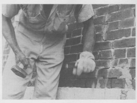
Fig. 4. The stonemason is demonstrating the proper way to cut out mortar joints. The use of a hammer and chisel is rather slow, but avoids the pitfalls of using a saw with a carborundum blade.
