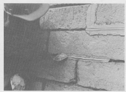
Fig. 7. The mason is "tooling the joint" with his pointing tool.
