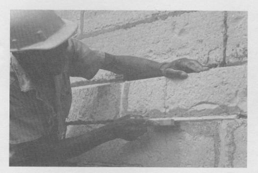
Fig. 9. In this final step in repointing the mason brushes off the mortar that remains on the face of the stone. The original joint that he is trying to approximate is flush with the edges of the stone and raised with a V-profile. The mortar in view above him is a midnineteenth - century replacement of the earlier type.
