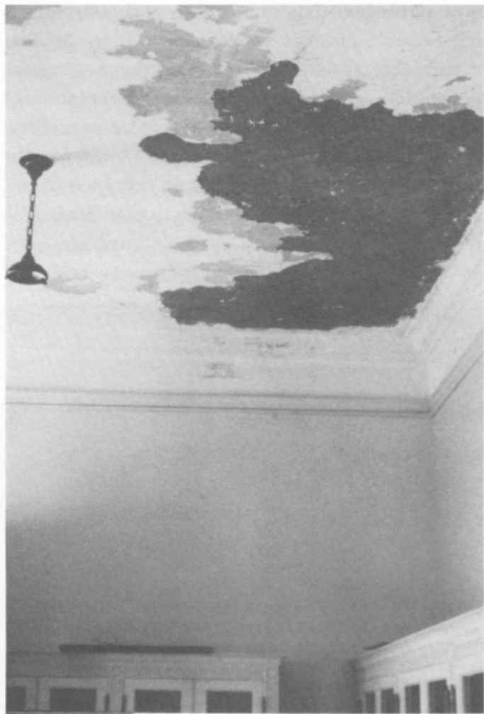
Problems inside usually mean problems outside. This damaged ceiling requires evaluation of the roof to determine what repairs are necessary. Photo courtesy of Northeast Document Conservation Center, Andover, Massachusetts.
