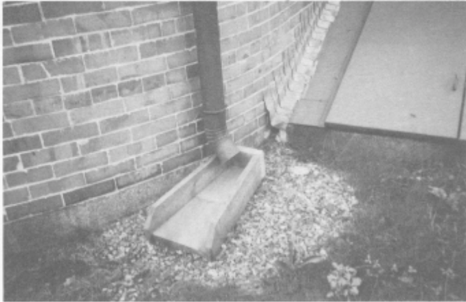
Historically appropriate drainage strategies are available for historic house museums. Note the wooden chute and the gravel bed used to reduce water in the basement of this nineteenth-century building. Photo courtesy of the Exeter Historical Society, Exeter, New Hampshire and Northeast Document Conservation Center, Andover, Massachusetts.
