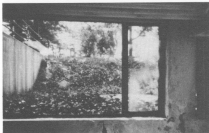
Damage on the inside of a building often means problems on the outside. The plaster deterioration at the window is from water flowing down the planted hill. Drains left out of the original design had to be installed later at a higher cost than they would have meant during construction. Photo courtesy of Northeast Document Conservation Center, Andover, Massachusetts.
