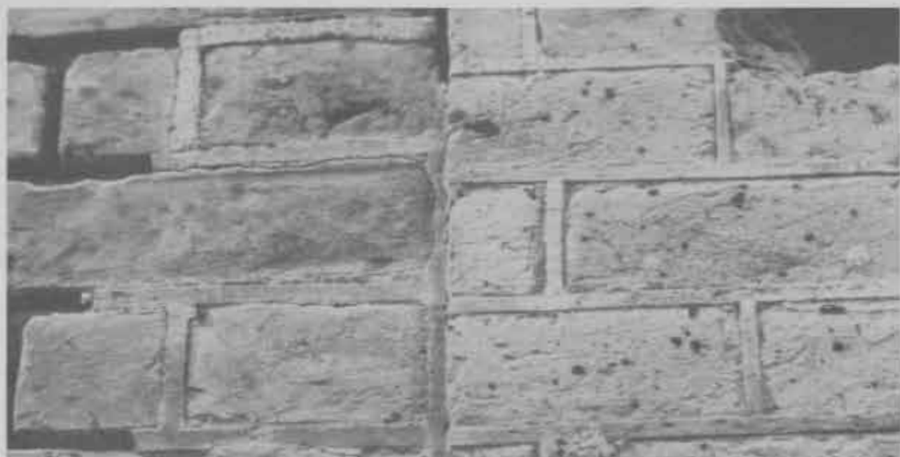
Off Key West, Florida, stands Fort Jefferson, built around 1846. The section of masonry shown above is the only remaining original brick work on the structure's exterior. The correct restoration of the original mortar tooling was made possible by the evidence shown in the structural brick arch to the left of the vertical joint and the decorative brick facing to the right.
