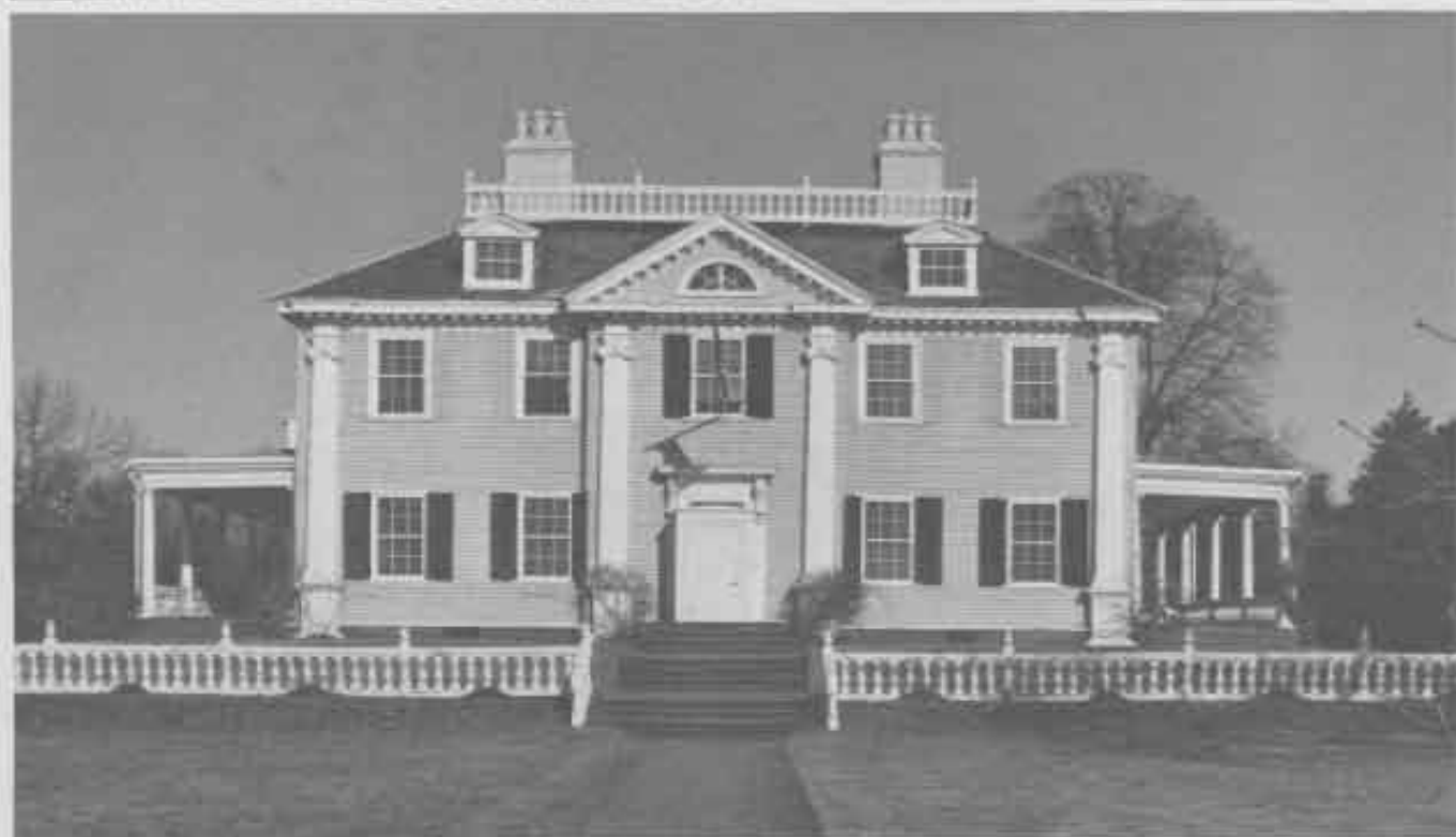
Top left: the left half of this house was constructed in the seventeenth century, and the right half was added in 1709 by the original owner. At that time, the windows in the original structure were changed to match those in the new addition. Top right: The windows in the original part of the house were restored to an earlier period than those in the later addition, thus, creating a house that never existed previously. Bottom: This house was constructed in 1759, and the porches were added in the 1790s. As important additions to the structure, the owners decided not to remove them when restoring the house.
