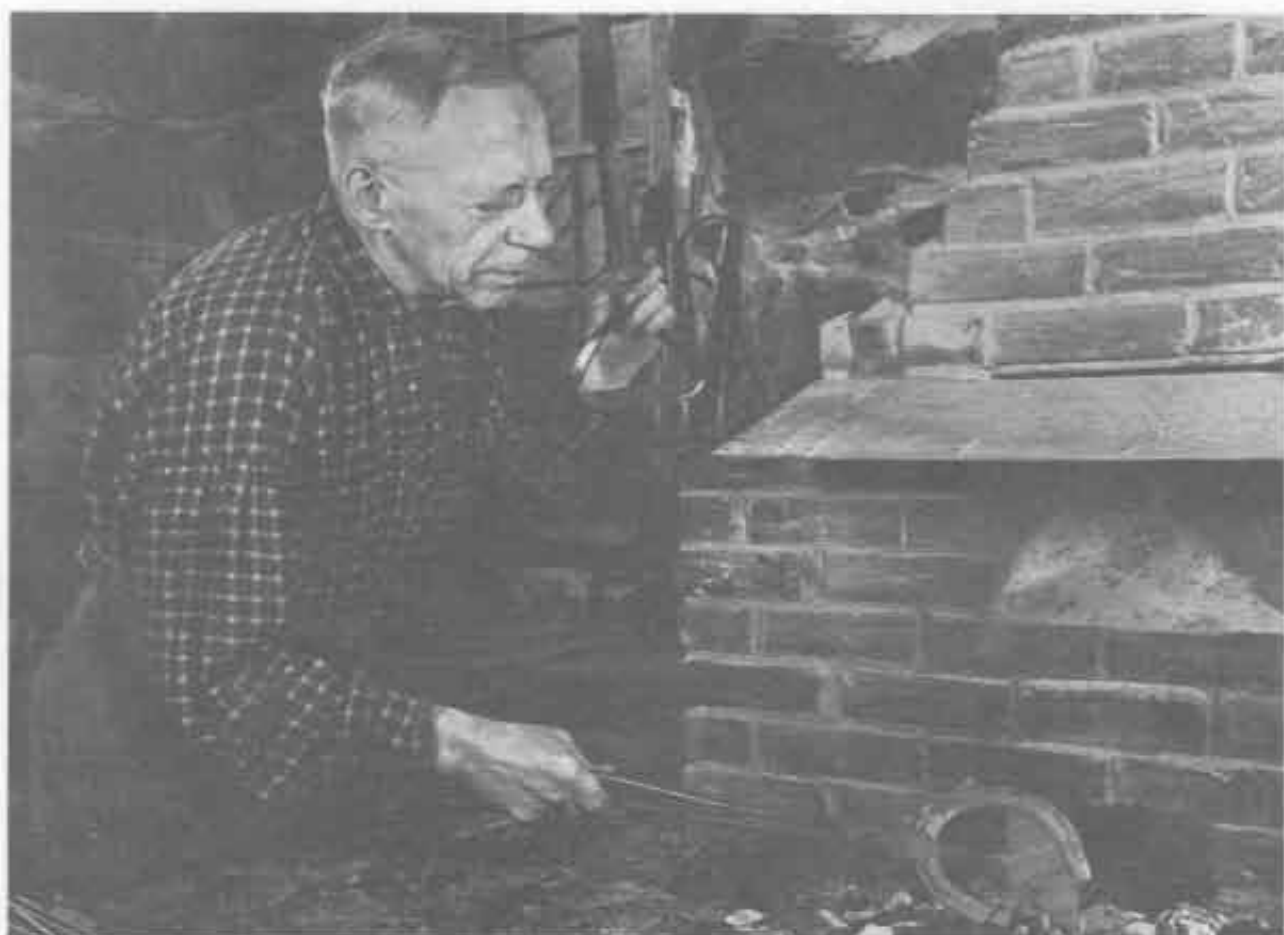
Hand-wrought nails were turned out at forges such as this two-man forge operated by a blacksmith at Old Sturbridge Village, Sturbridge, Massachusetts. Latches, hinges, candlestands, foot scrapers, toasting forks, and a myriad of other objects were made by smiths at these forges of yesteryear. (Photo: Old Sturbridge Village.)
