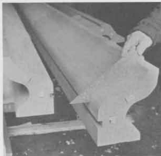
A metal template is used to gauge the accuracy of a wooden cornice replacement.
