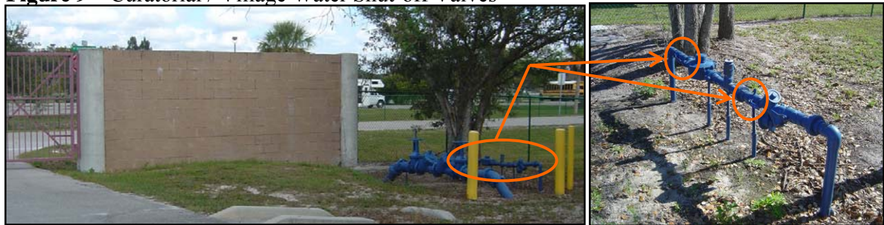
Figure 9 – Curatorial / Village Water Shut-off Valves
